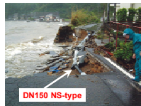
Japan NS-type DIP in typhoon (courtesy Prof. Miyajima)
