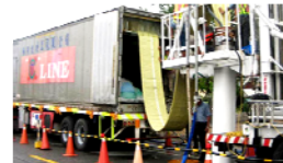
Plastics piping system (hose lining) for renovation in Taipei (courtesy Ashimori Industry Co.)
