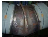
Steel pipe for crossing fault (SPF) using buckling pattern (courtesy JFE Engineering)
